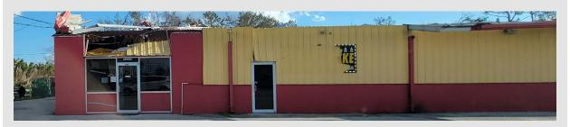
This auto body shop in Port Charlotte experienced severe damage to the siding and roof. The old metal panel siding was poorly connected to the wall and roof.
