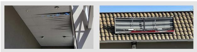
Damage to exterior ceiling panels caused by local wind gust effects in a long corridor (left) and damaged sign (right).
