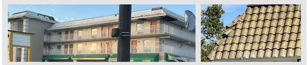
Some older commercial properties sustained significant tile roof damage. The roof type on these buildings is similar to a flat roof, which causes high suction pressures on the tiles in the corners. Ridges are often the weaker parts of roofs because of higher suction pressures compared to other roof areas.
