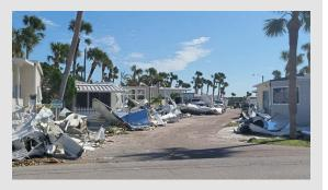
Large amounts of debris from damaged attached structures and other building components from manufactured homes increase the risk of damage to neighboring homes.
