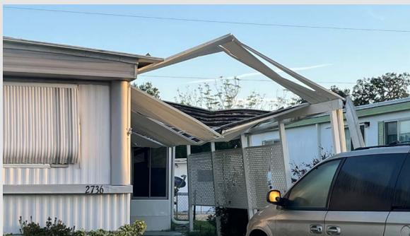
In Category 2 wind speeds, attached structures, such as carports are vulnerable and can get torn off, causing progressive damage to the main buildings.
