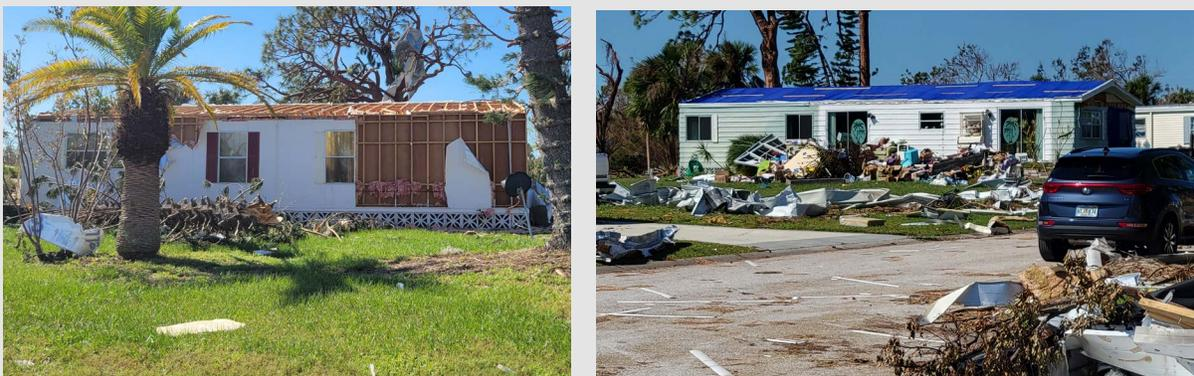
**Manufactured homes in Englewood sustained extensive interior damage due to water infiltration from exposed roofs and walls when the roof cover and wall siding were damaged by high winds.**
