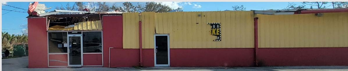
**This auto body shop in Port Charlotte experienced severe damage to the siding and roof. The old metal panel siding was poorly connected to the wall and roof.**
