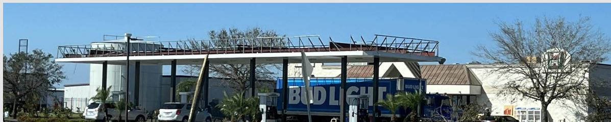
**Gas station pavilions sustained heavy damage from wind uplift due to their light weight and large surface area.**
