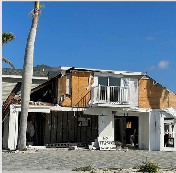
Wind damaged the roof structures of single-family homes in Fort Myers Beach, which led to progressive damage to the wall structures and total losses in many cases.
