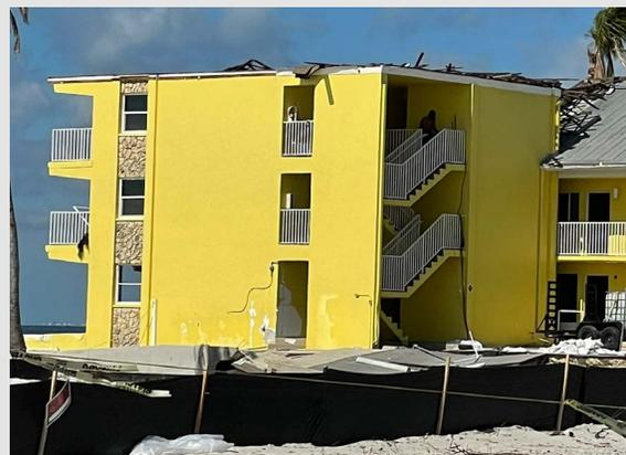
Wind peeled the metal roof of a public building from its rafters (left) and sheared the metal roof completely off a multifamily building (right).
