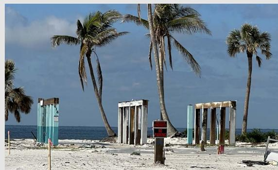
The buildings on the left have higher first-floor heights and stronger foundation connections, which left them undamaged by the storm surge while nearby homes were swept away (as shown by the piles left behind in the foreground, circled in red). The photo on the right shows piles left behind by a building with a lower first-floor height and poor foundation connections, which made it vulnerable to storm surge and led to the entire building being swept away.
