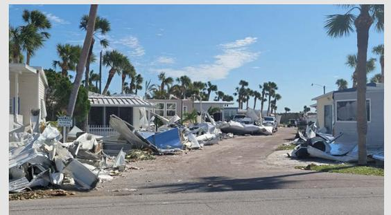
Large amounts of debris from damaged attached structures and other building components from manufactured homes increase the risk of damage to neighboring homes.
