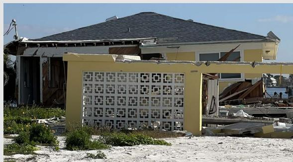
This home in Fort Myers Beach (shown before Ian on the left and after on the right) was shifted off its foundation due to storm surge and sustained extensive structural damage leading to a total loss. Not only did the foundation connection fail, but the foundation itself partially collapsed because it was a relatively old building (built in 1952).
