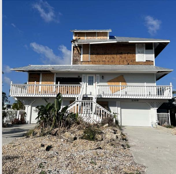
The detachment of roof components is the most common reason for a loss of structural integrity due to high winds. These Pine Island homes were built before the first wind engineering based design requirements, so the wind speeds from Hurricane Ian exceeded the design wind speeds.
