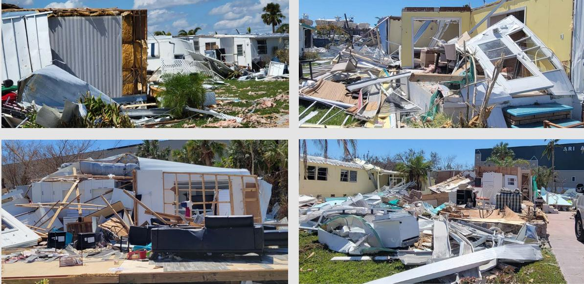
**Many manufactured homes in Placida were completely destroyed with detached roofs and collapsed walls.**
