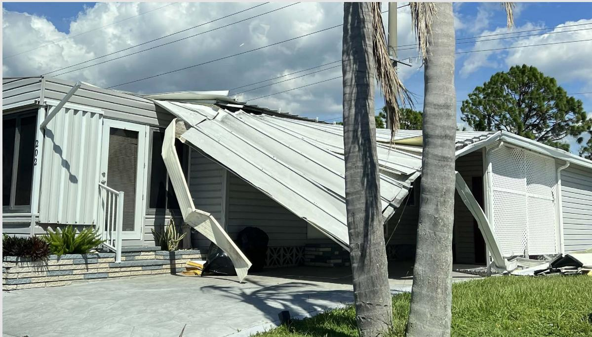
This manufactured home lost part of its roof after an attached structure was damaged.
