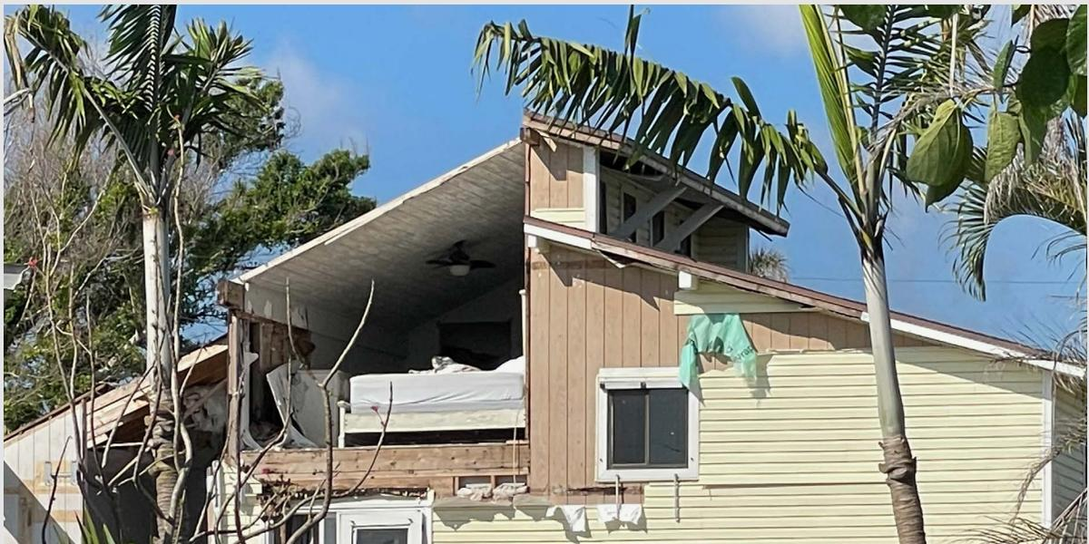
Extreme structural damage to the wood frame wall of this Pine Island home led to severe interior damage. Damaged windows and breaches on the gable caused higher pressure on the roof and wall. The wall structure in this building collapsed even before the roof structure failed.
