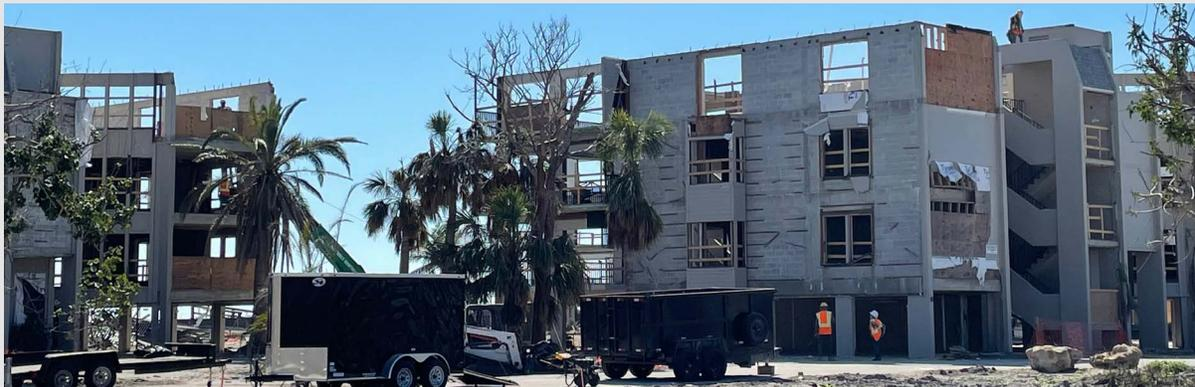
The flat wooden roofs on these multifamily residences were compromised, which increased the pressure on openings and walls and caused them to fail. Once the building envelope is compromised, wind and water can fully damage the interior, resulting in a total loss.
