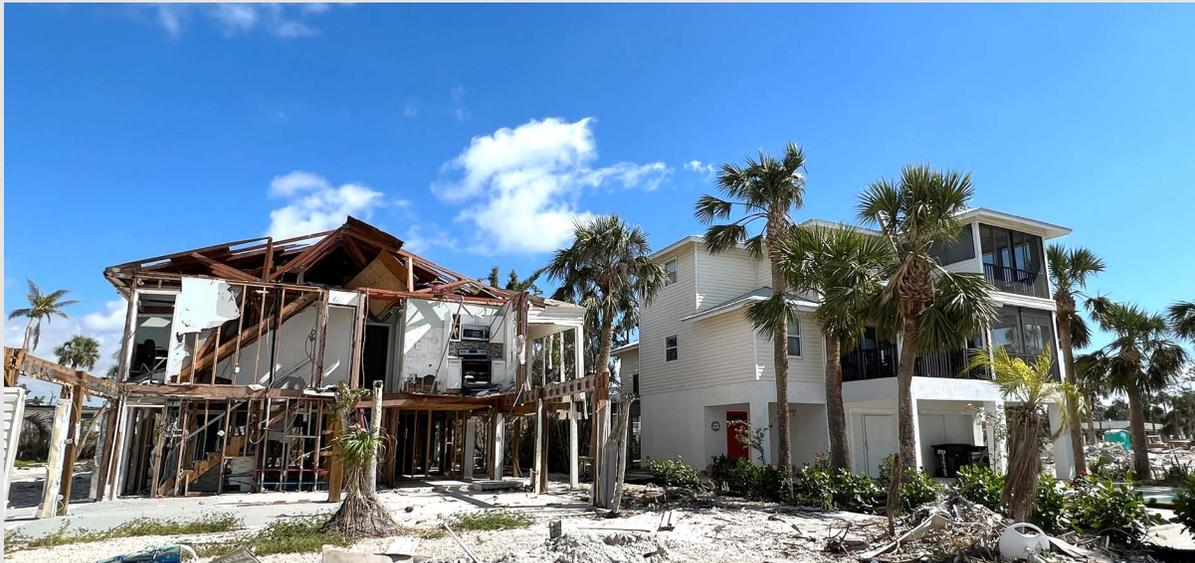
The home on the left was constructed of wood frame with a shingle roof in 1972, while the home on the right was constructed of masonry with a metal roof in 1997. The wood frame home was completely destroyed, while the masonry home sustained only minor screen damage and water leakage.
