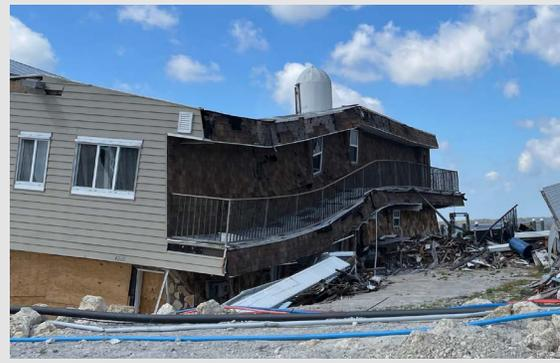
**Storm surge can cause a failure of the foundation connection and foundation of coastal buildings, resulting in total losses. These homes were built on solid wall foundations, which failed due to storm surge.**
