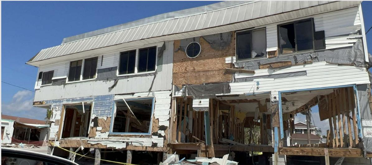
This building on Fort Myers Beach has a first floor that is about four feet above ground level, but the storm surge in this location was twelve feet, which led to storm surge damage on the first-floor structure and extensive interior losses. In addition to the surge damage, the second-floor wall siding and openings were severely damaged by high winds.
