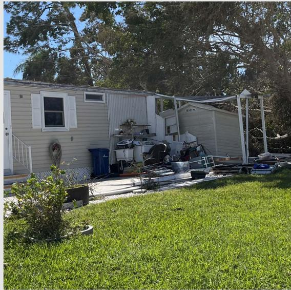
The attached structures of these manufactured homes were lifted up from pressure below the structure. Because these structures are connected to the roof, parts of the roof are also progressively damaged, first because of wind-induced vibration and then because of full lift off of the attached structure.
