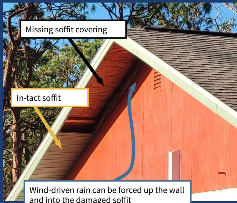
Soffit damage can necessitate complete replacement of a building's siding because wind-driven rain gets under the siding and into the walls. Rainwater can also be driven over the exterior wall into wall breaches and attic spaces. Water infiltration can then lead to significant interior damage, increasing the ultimate loss.
