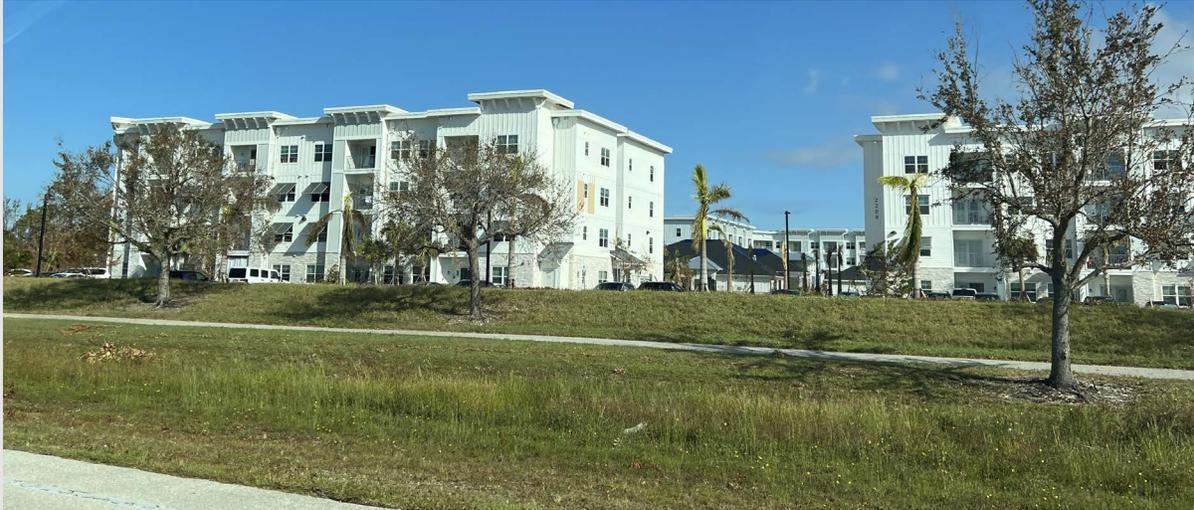
**A multifamily residential structure in Cape Coral appears undamaged. The roof of this building is a built-up wood deck system, which is much more wind-resistant than tile.**
