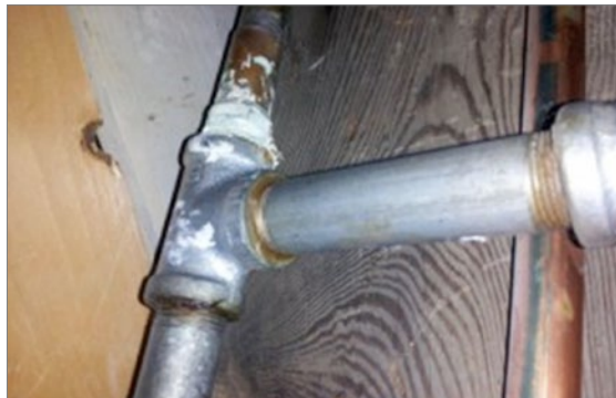
Fig. 2. Corrosion on Galvanized Steel Piping Photo courtesy Levco Builders.
